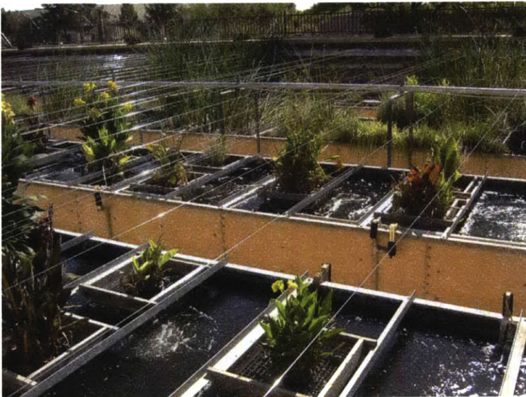
Ethel M. Chocolate's industrial wastewater treatment living machine in Henderson, Nevada.
