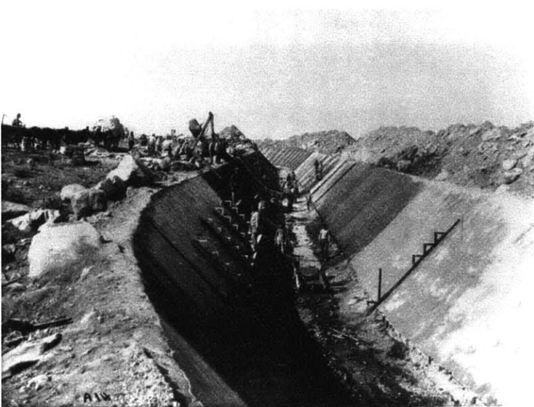
Placing concrete in the open channel. Photo from the LADWP archives.
