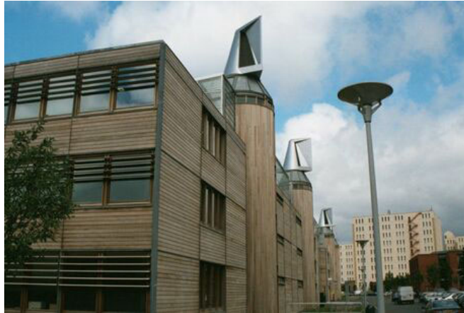
Figure 30. Stacks facilitate airflow in this naturally ventilated building at Nottingham University's campus in the United Kingdom. (Photograph by Brian Dean)
