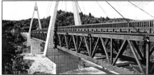
Figure 1 – Glulam bridge (courtesy of APA: The Engineered Wood Association)
