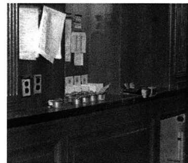
Pneumatic tubes deliver call slips to the Main Reading Room where they are sorted and sent to all 8 levels of the underground stacks.
