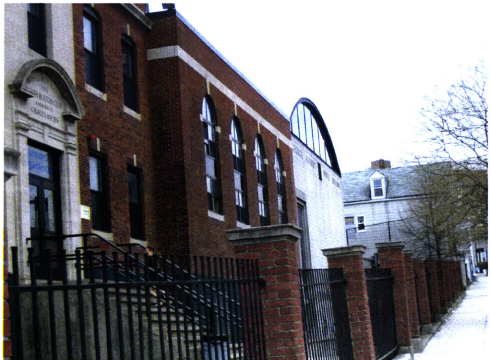
Figure 3-e1: The front entrance to the South Boston BGC
