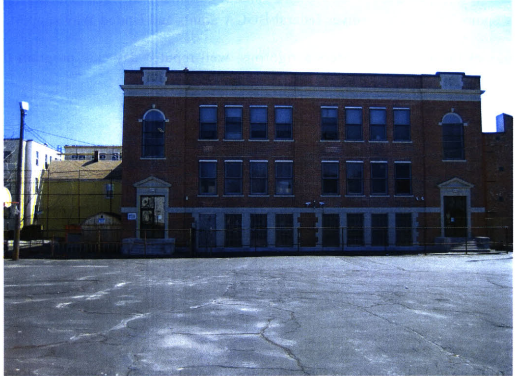
Figure 5g: The front façade of the Salesian East Boston BGC
