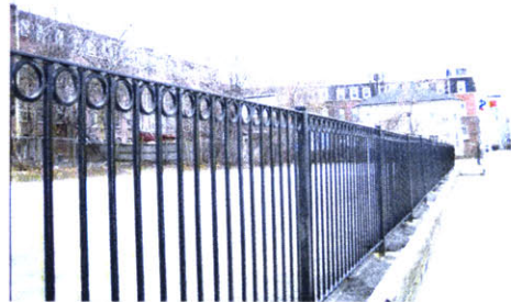
Figure 3-f8, right: The fence perimeter around the outdoor basketball court
