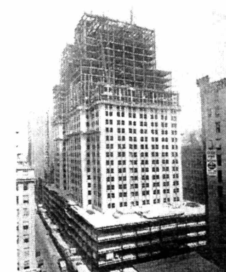
Figure 2.14: Empire State Building
