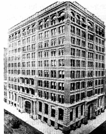
Figure 2.1: Home Insurance Building
