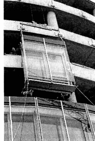
Figure 8.27: DSF Construction Unit
