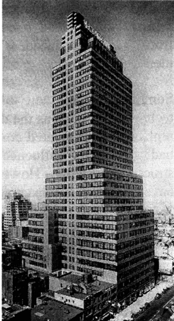
Figure 2.27: McGraw Hill Building
