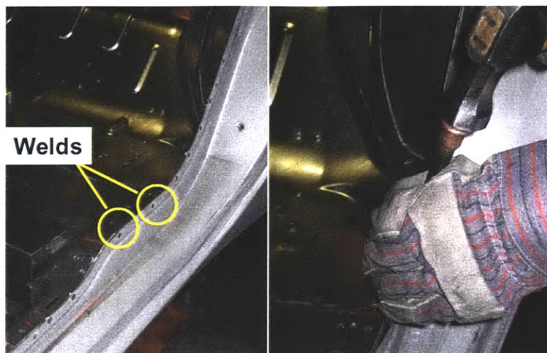
Figure 7. Chisel Check Performed on Welds
