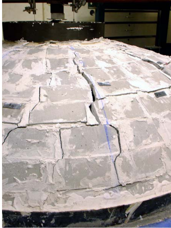
Figure 6.10. Dome I: Cracks in the hoop direction, or hinge circles, created the collapse mechanism after displacement exceeded 0.5 in.
