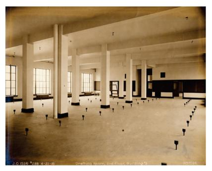
**Fig. 100:** Photo taken during construction of former Building 3, and revealing the legibility of the structural system of the first type of stem.
