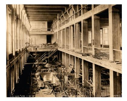
**Fig. 99:** Photo taken during construction of former Building 7, and revealing the legibility of the structural system of the second type of stem.
