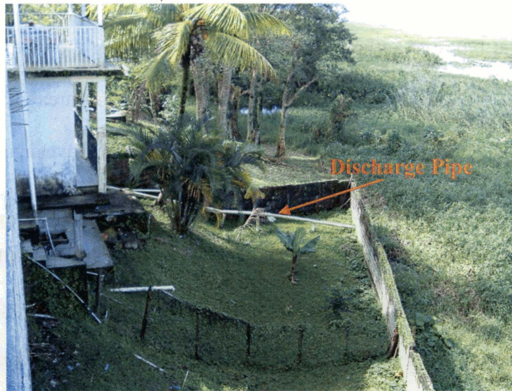
Figure 4.6: Discharge pipe from La Casetas
