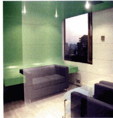
The green lackered finish was done on site after all modules were assembled and hunged. Images by the author.
