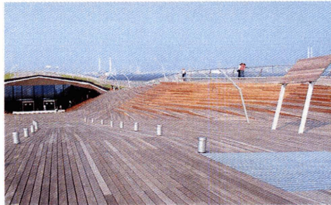
Figure 16 and figure 17 The smooth continuous surface of the Yokohama Port project, built as a faceted set of planar surfaces restricted by the material used. The curved
