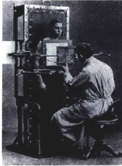
Figure 2.3: Radiographic system using fluorescent screen. [Image taken from Imaginis, 2006]
