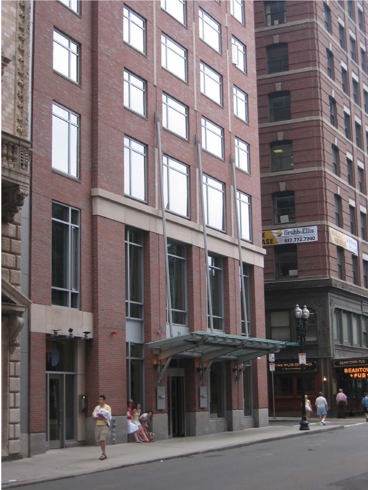
Nine Zero, a newly constructed boutique hotel located in Boston.
