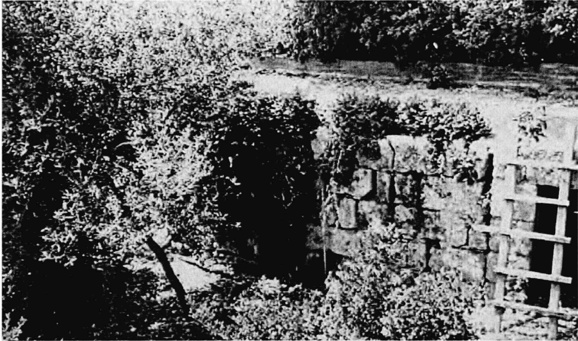
Figure 33 Retaining wall of upper terrace, al-Rummaniya
