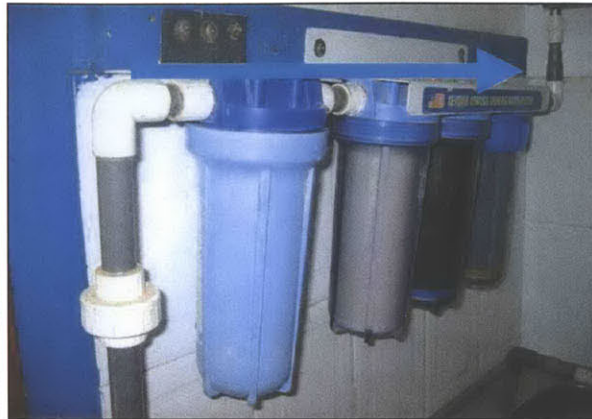
Figure 6.6: Series of yarn, fiber, granular carbon and carbon matrix filters. Arrow shows flow direction
