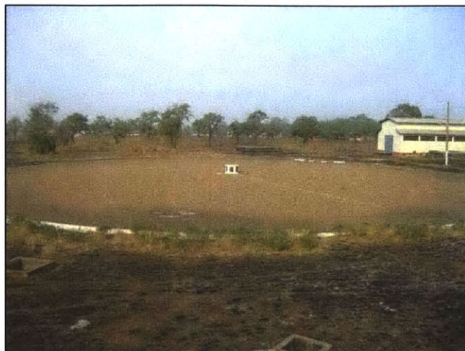
Figure 5.18: The treated water is stored in under-ground tanks (perimeter marked by white painted stones) prior to pumping into the distribution pipes to homes and businesses
