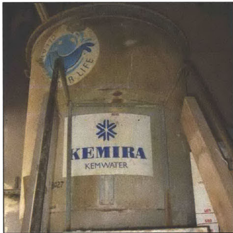
Figure 5.4: Aluminium sulfate solution
