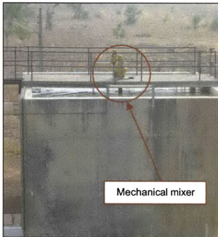
Figure 5.7: Flocculation/ coagulation chamber with mechanical mixer suspended on a horizontal shaft
