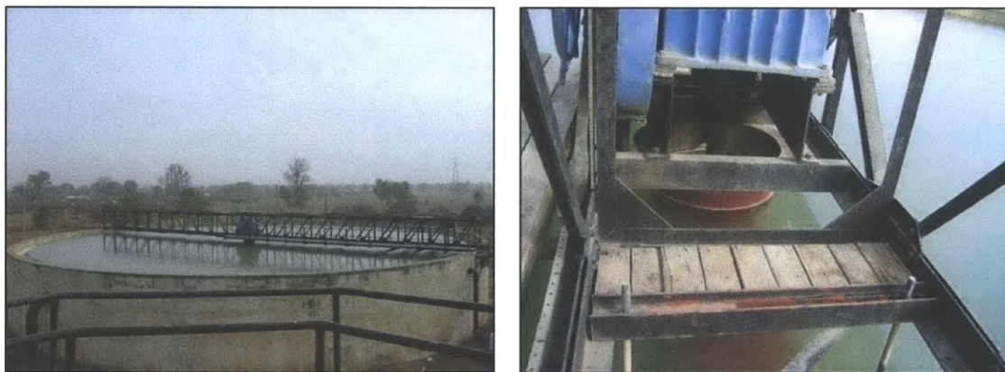
Figure 5.10: Sedimentation tanks showing inlet well and drive
