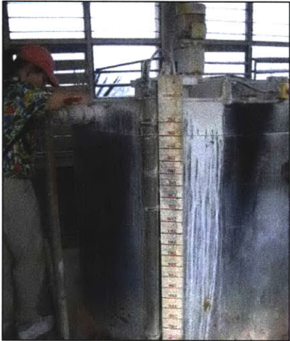
Figure 5.16: Handling tanks mix and meter lime
