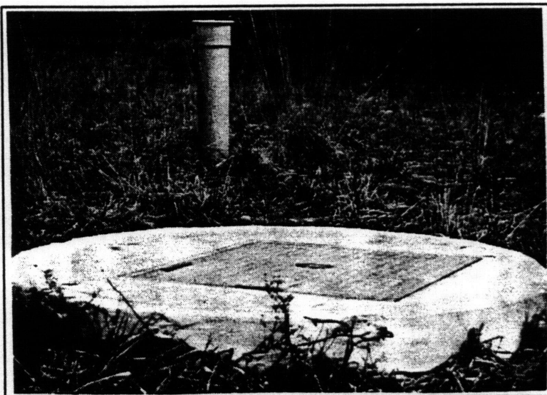
An unobstrusive data collection vault for one of the groundwater extraction wells at CS-4. An observation test well is located behind the vault and is periodically sampled to help evaluate the extraction system's performance. Such test wells can easily be installed as a flush-mount well, which will be the plan for off-base installations associated with the six plume containment project.
