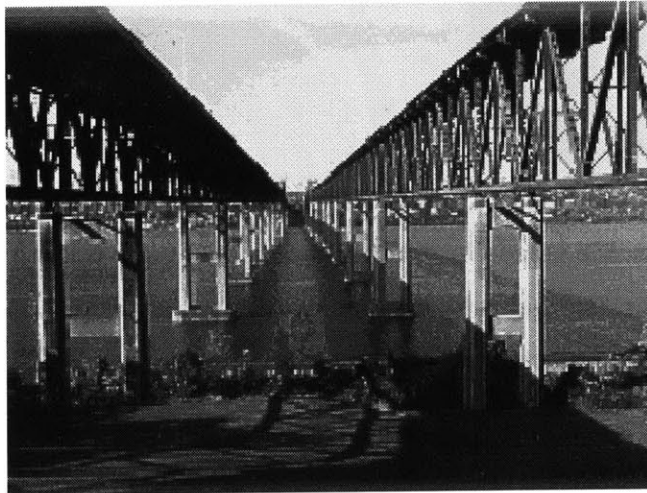
Figure 1.2. Twin structures for the Newburgh-Beacon Crossings of the Hudson River, built in 1962 and 1971 with almost identical cantilevered truss form (NYSBA, www.nysba.state.ny.us )
