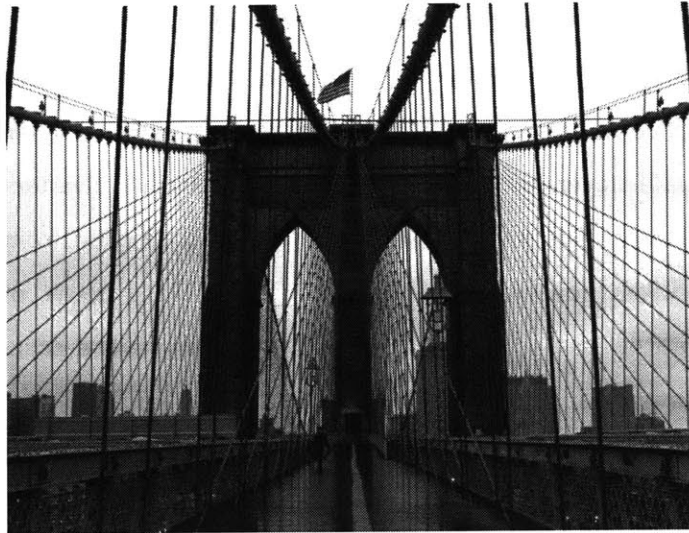
Figure 2. Cable-stayed suspension bridge, Brooklyn Bridge, 1883, NY (Nikolas Jansberg)
