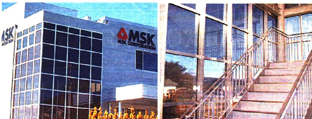
Figure 6-2 – Amorphous Si PV panels used in BIPV application (courtesy Kaneka Silicon)
