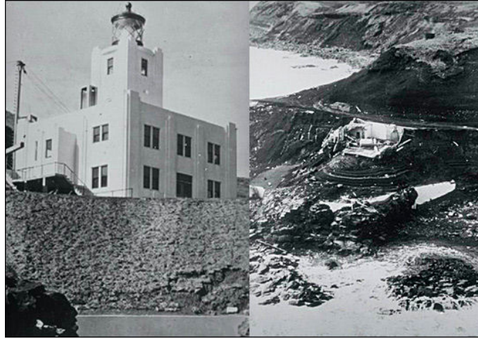
Figure 3.3.1: The Scotch Cap lighthouse on Unimak Island, Alaska before and after the 1946 tsunami [University of Washington, 2005].
