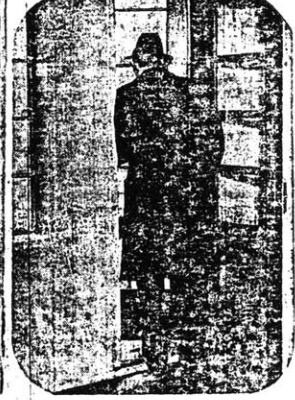
A man weighing 175 pounds wedges in this 18-inch door as he tries to go onto the porch from the living room—and that is the only way to get on the porch unless he climbs up from the ground on a ladder.
