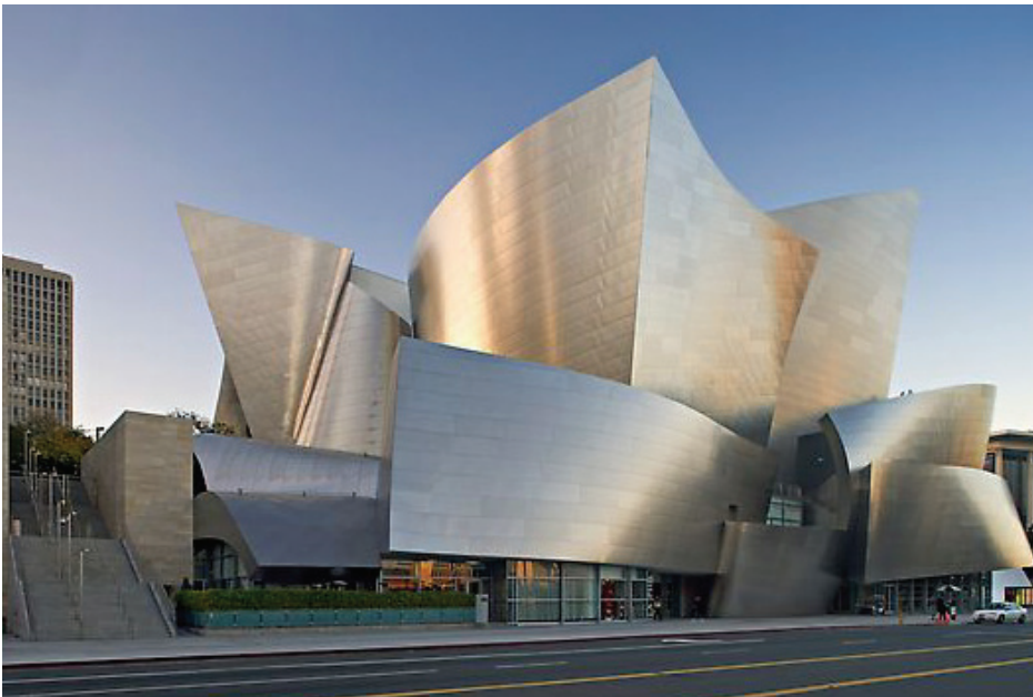
figure 2.10: Walt Disney Concert Hall, Los Angeles, CA, USA, designed by Frank Gehry. www.terrageria.com
