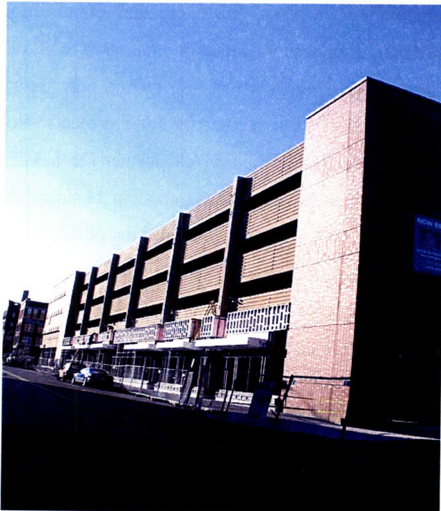
JAM parking garage going up across Jackson Street
