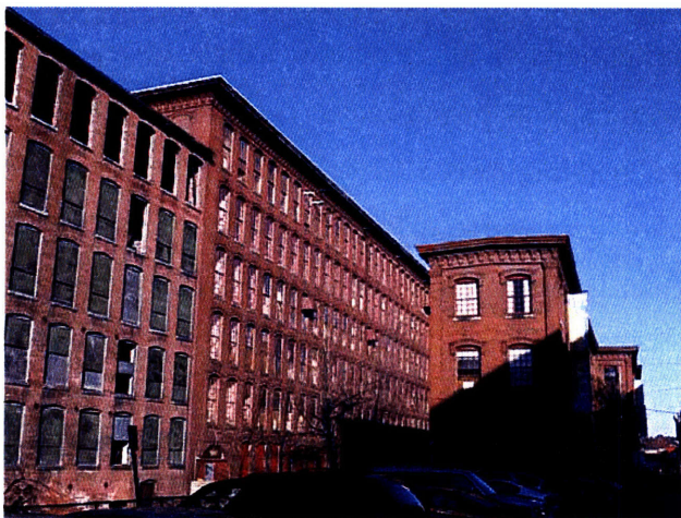
CMAA- Courier Building on Jackson Street
