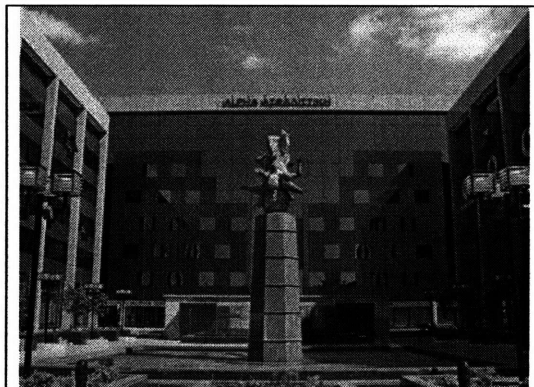
The Telco Facility
