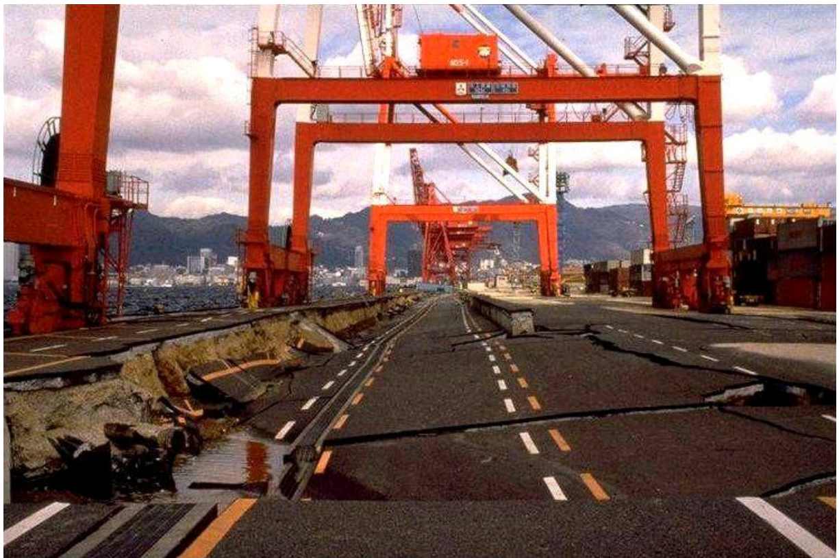
Figure 1-1 Significant damage in the Kobe port facilities due to the 1995 Kobe earthquake
