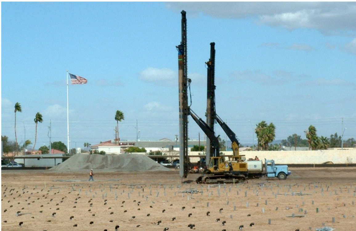
Figure 1-3 Installation of PV drains (Ellington Cross)
