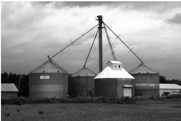
A private farm elevator near Aurora, Nebraska, comprised of augers and grain bins. July, 2008. Photographed by author.
