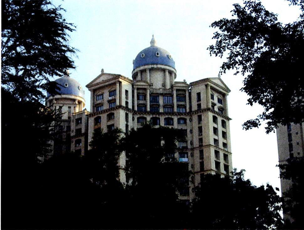
Fig. 11: Apartment Tower at Hiranandani Complex, Powai designed by Hafeez Contractor indicating the neo-Baroque domes (Online source: http://www.flickr.com/photos/himanshu_sarpotdar/358027190/ )
