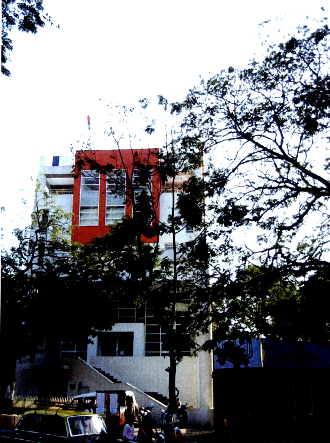
Fig. 18: Street view of The Diamond Jubilee High School
