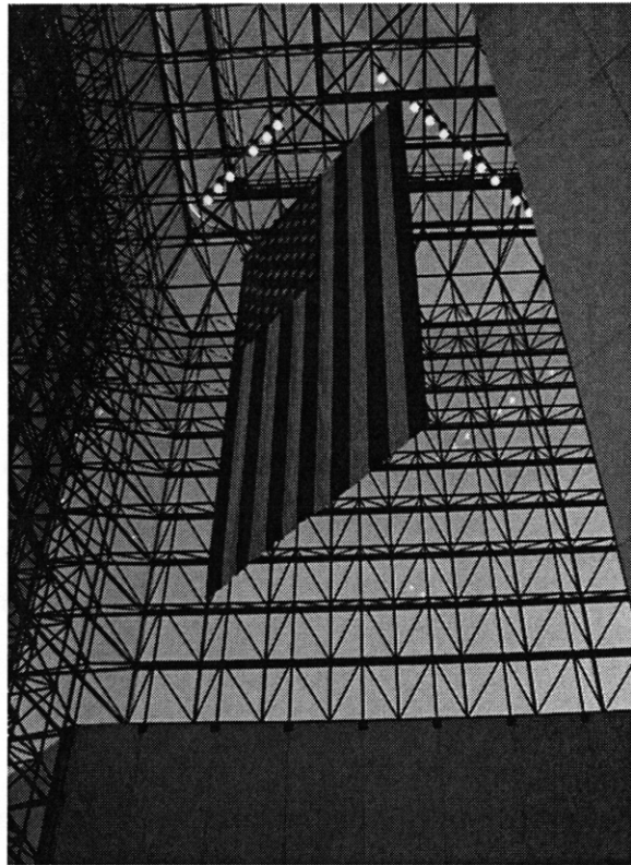
1.1 Atrium at the John F. Kennedy Library, South Boston, Massachusetts (Photo by Author © 2004).
