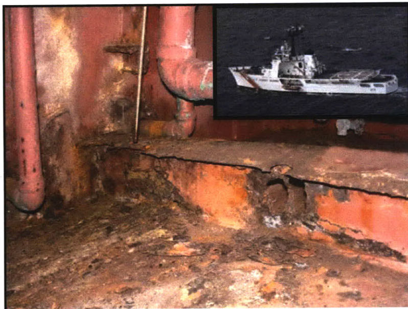
Severe corrosion requiring emergency drydock of the 40 year old Cutter VALIANT
