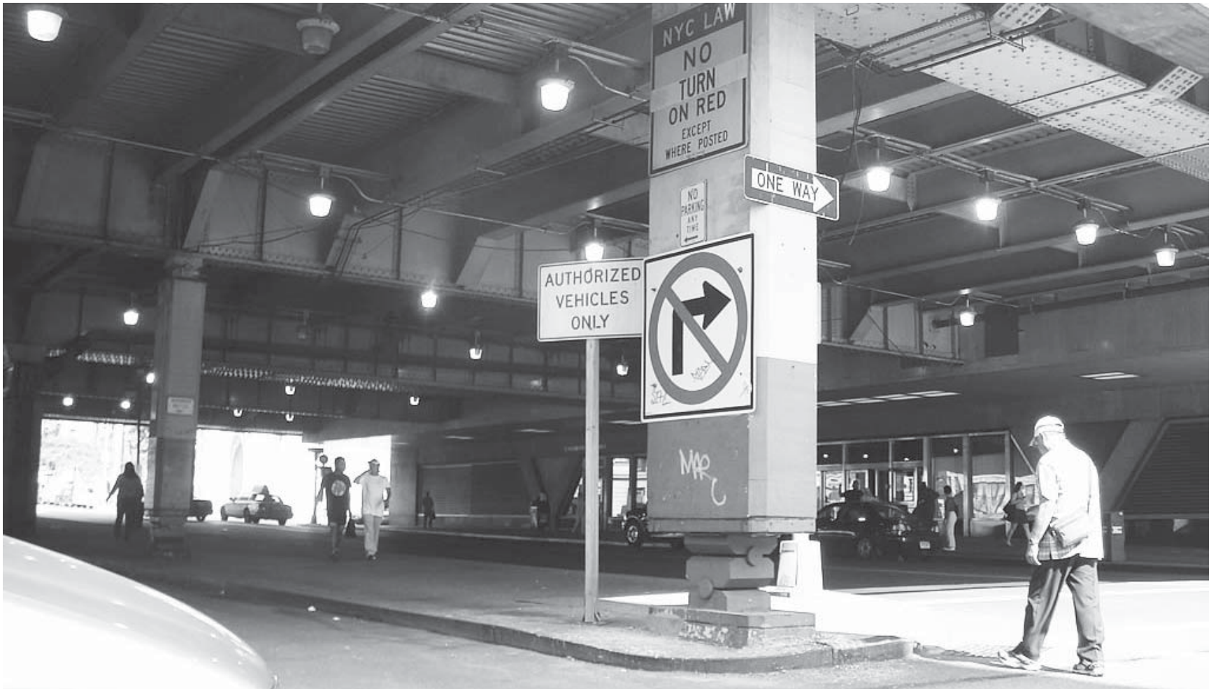
EXISTING FORT WASHINGTON AVENUE BUS TERMINAL ENTRANCE
