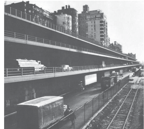
BROOKLYN-QUEENS EXPRESSWAY, NEW YORK
