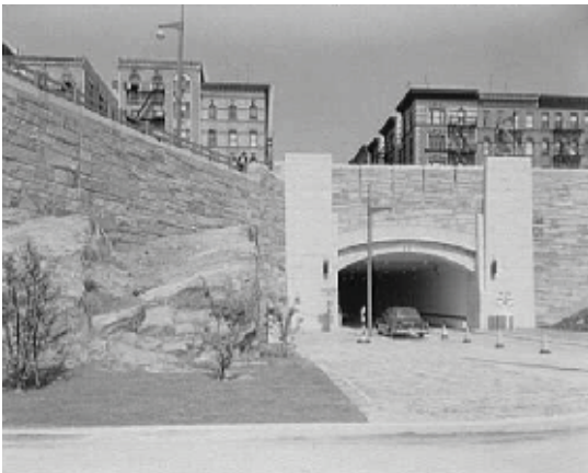
178TH STREET TUNNEL
