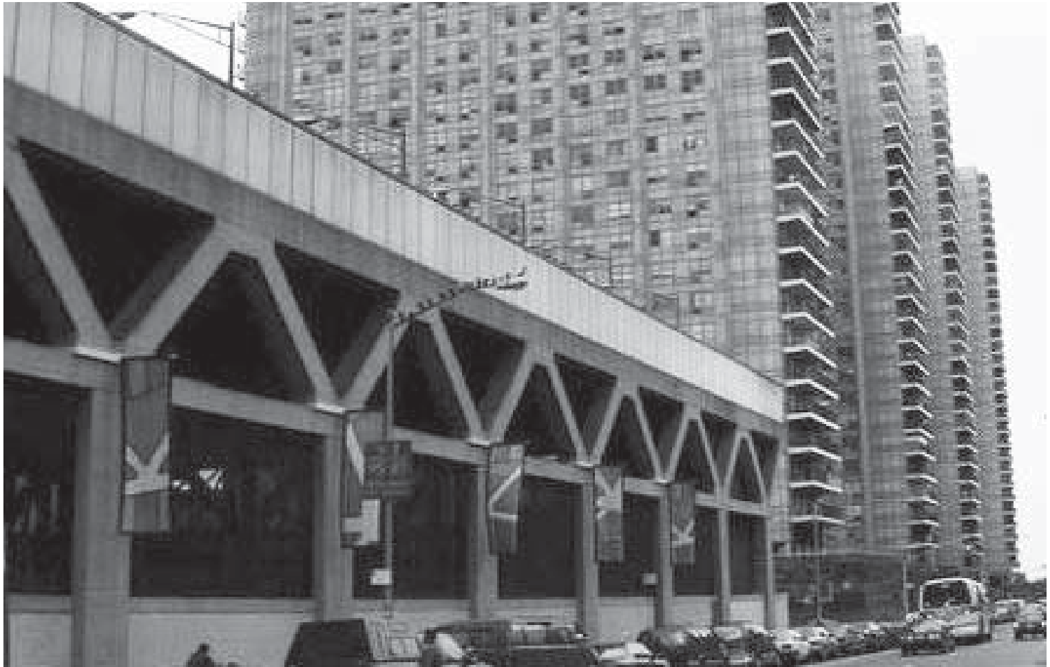
HOLLOW PARKING STRUCTURE AND WASHINGTON BRIDGE APARTMENTS
