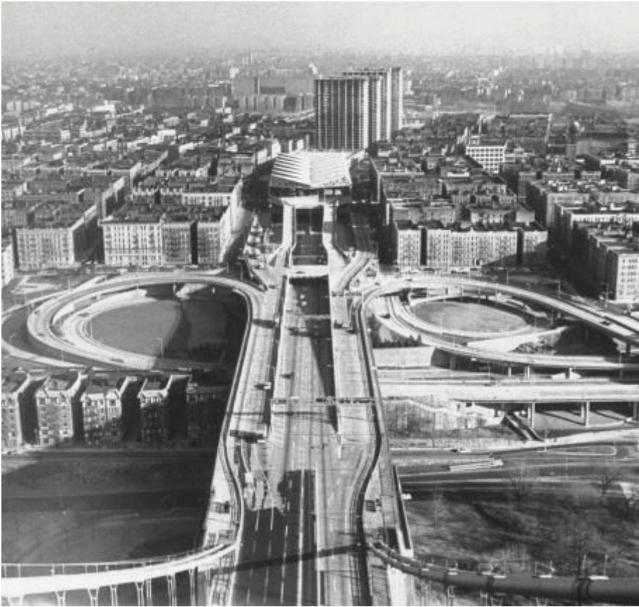
GEORGE WASHINGTON BRIDGE BUS TERMINAL WASHINGTON HEIGHTS, NEW YORK
