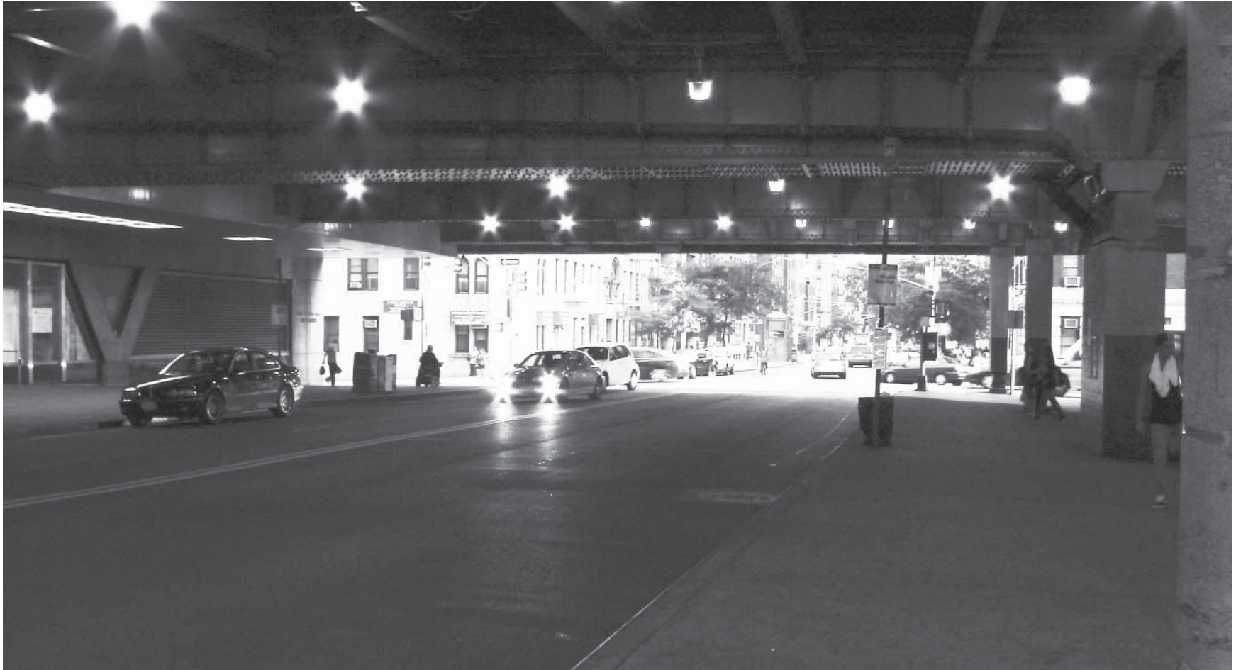
FORT WASHINGTON AVENUE ENTRANCE
