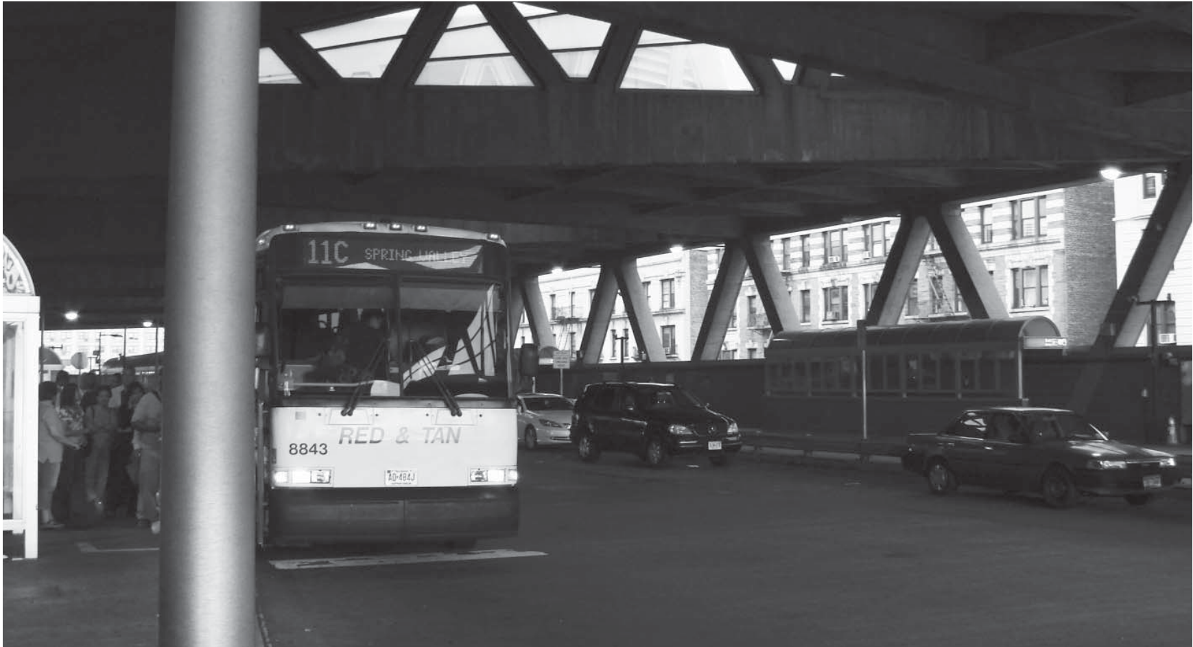
DARK BUS TERMINAL LEVEL
