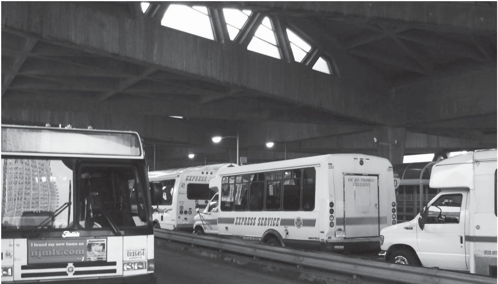
EXISTING GEORGE WASHINGTON BRIDGE BUS TERMINAL INTERIOR
