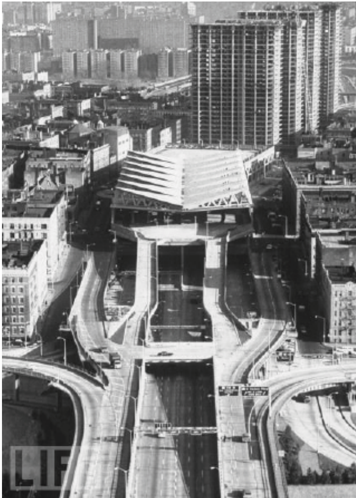
BUS TERMINAL AND WASHINGTON APARTMENT CONSTRUCTION
