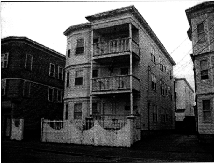
Figure 1: Typical "Triple Decker" in Lawrence neighborhood.
