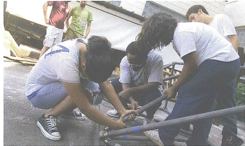
Students assemble the space truss. No instructions were provided yet they were able to put it together with minimal intervention.
