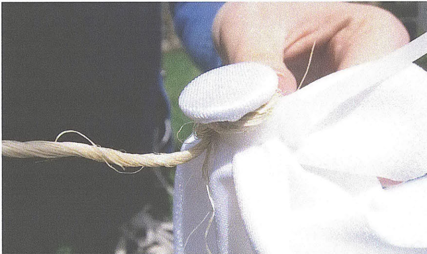
The construction method used to make The Microdot's Spandex tents requires minimal tools and results in easily-transformed, transformative spaces. Nylon zip ties enclosing ordinary pennies create structural connection nodes and bamboo poles elevate the fabric canopy.
