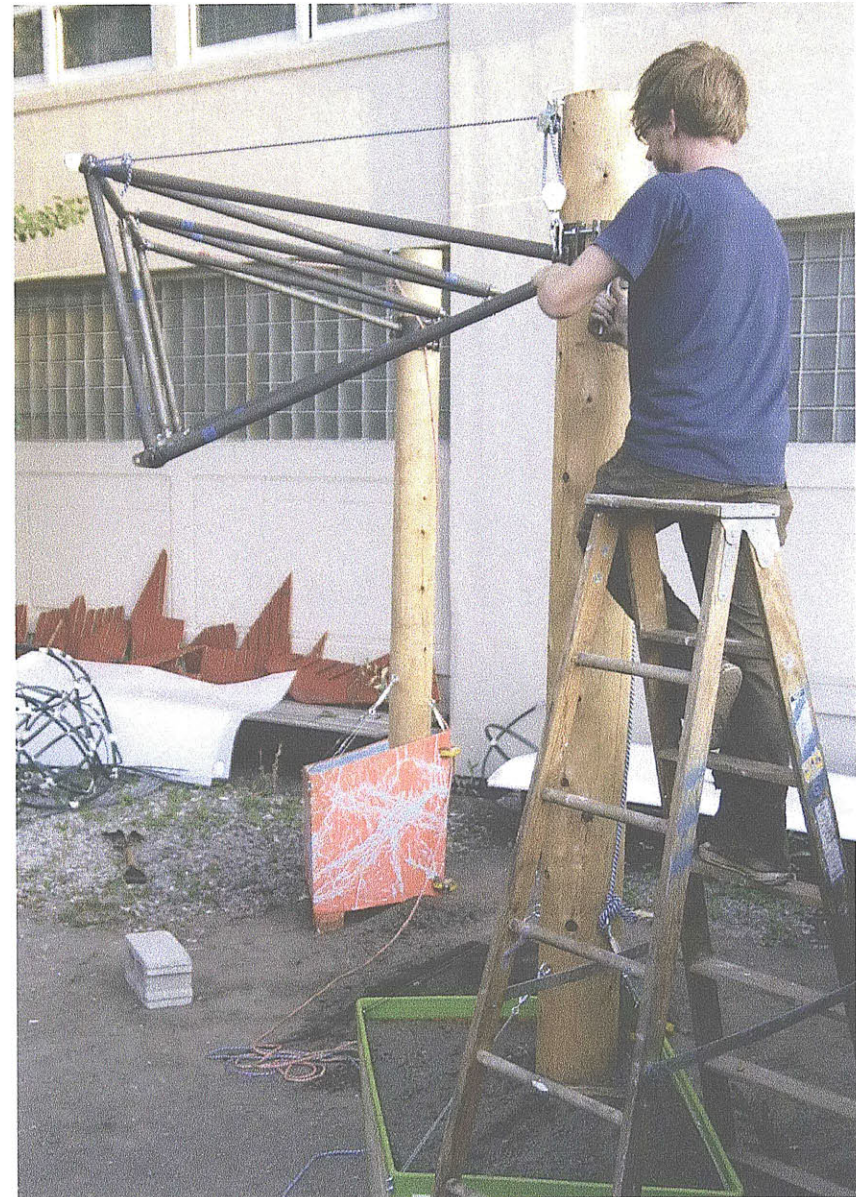
Bill demonstrates part of the module assembly process.
