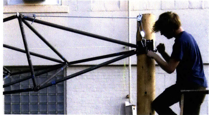
Bill raises a portion of the ring truss into place with a simple system of pulleys and ropes. Collars made from large-diameter pipes split in half guide the truss up the timber column. At the proper height, the bolts on the collar are tightened, clamping the truss in place.
