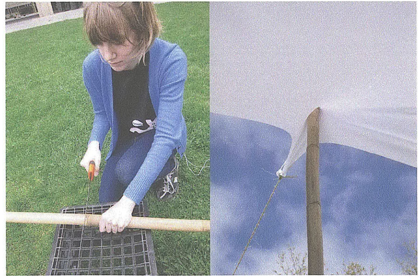
The construction method used to make The Microdot's Spandex tents requires minimal tools and results in easily-transformed, transformative spaces. Nylon zip ties enclosing ordinary pennies create structural connection nodes and bamboo poles elevate the fabric canopy.
