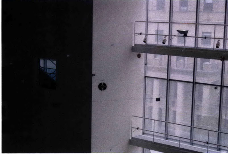
Figure 2.3: Sensors deployed in the atrium of E14.
