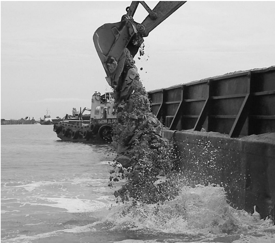
Figure 3-1: Photograph of a back hoe type dredge, which is an example of a point release (photo: Z. Huang, 2009).
