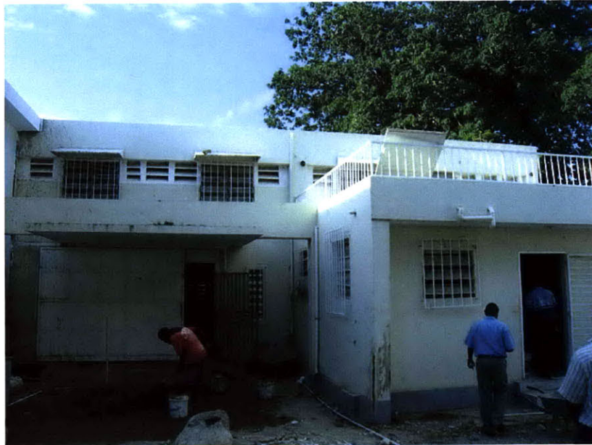
Figure 23: Exterior of the St. Marc Warehouse (during construction)
