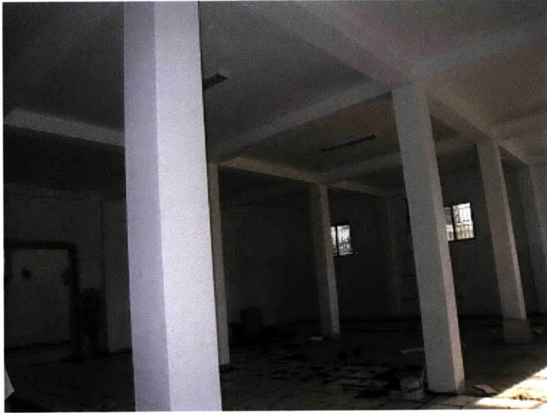
Figure 24: Interior of the St. Marc warehouse (during construction) Source: PIH Picasa Web Albums-ZL
