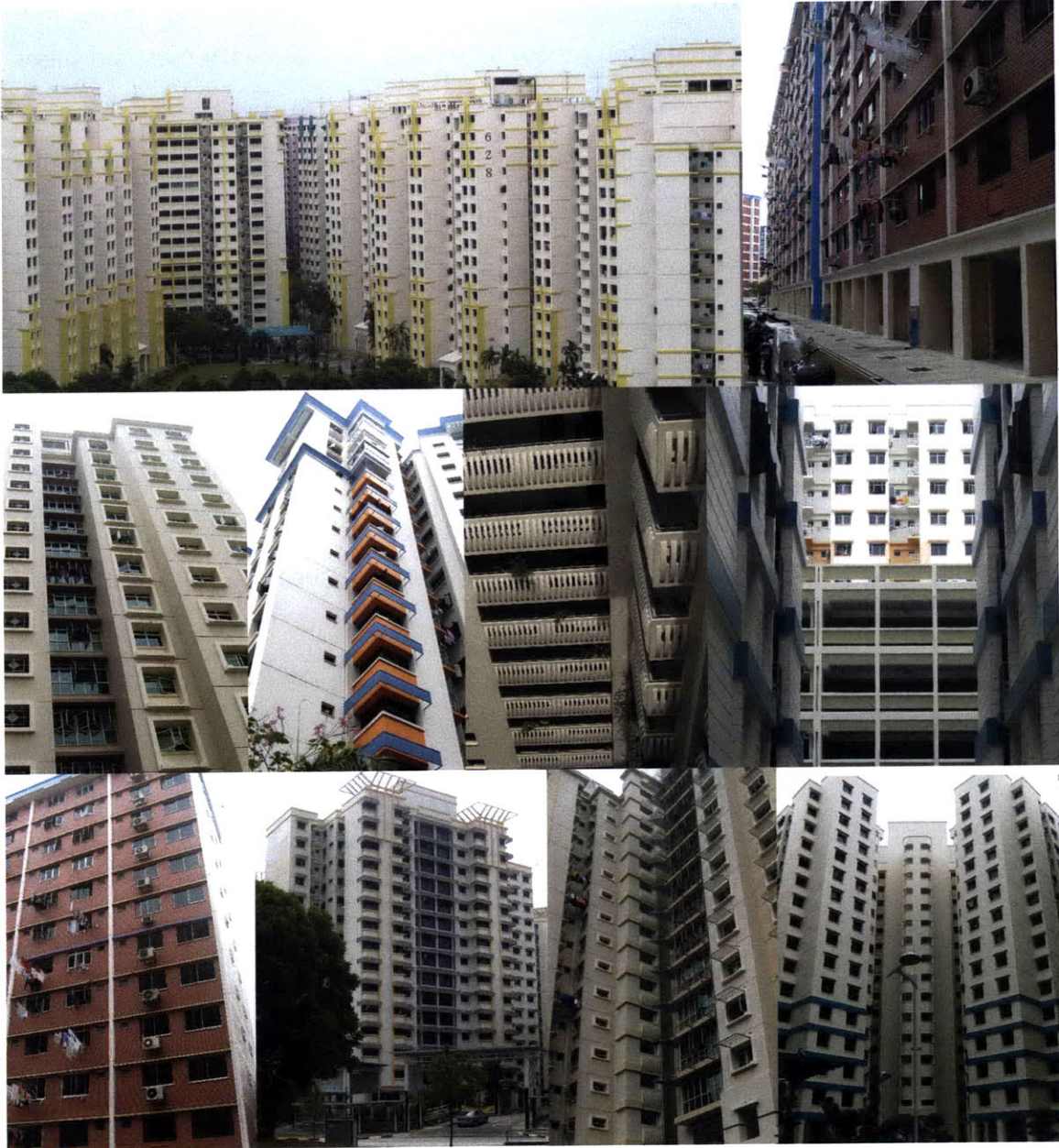
Figure 4-1: Building façades in Singapore with roughness elements
