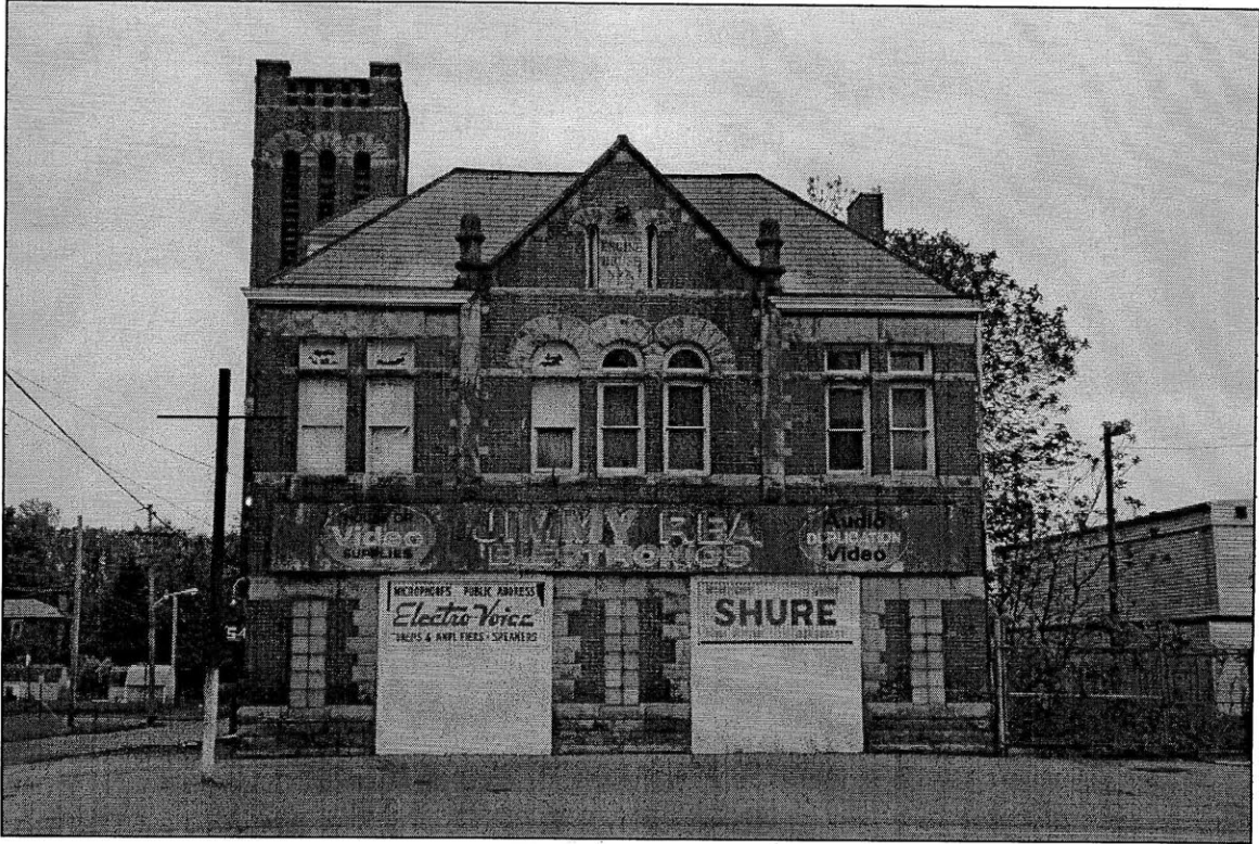
Abandoned building, West Broad Street, "the Bottoms," Columbus, Ohio, April 2010.
