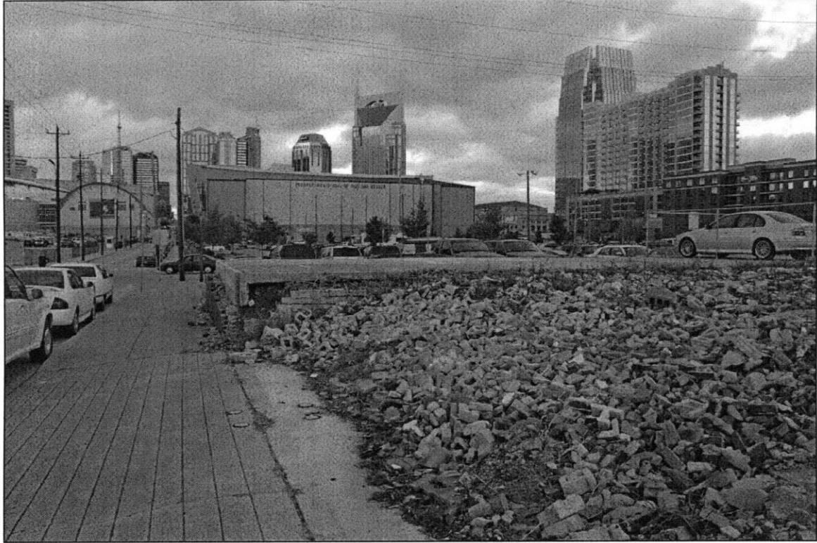
Demolition at the heart of SoBro (formerly Black Bottom) to clear the way for the new Music City convention center, Nashville, Tennessee, October 2009.
