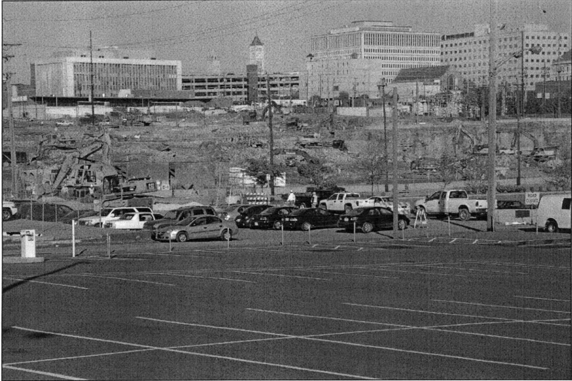
Music City convention center under construction in SoBro (formerly Black Bottom), Nashville, Tennessee, April 2010.
