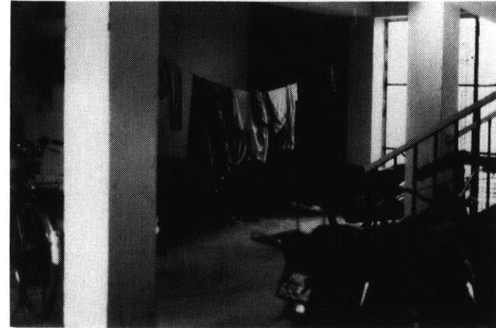
53. The semi-enclosed common space in each floor in front of the entrance to the units.
