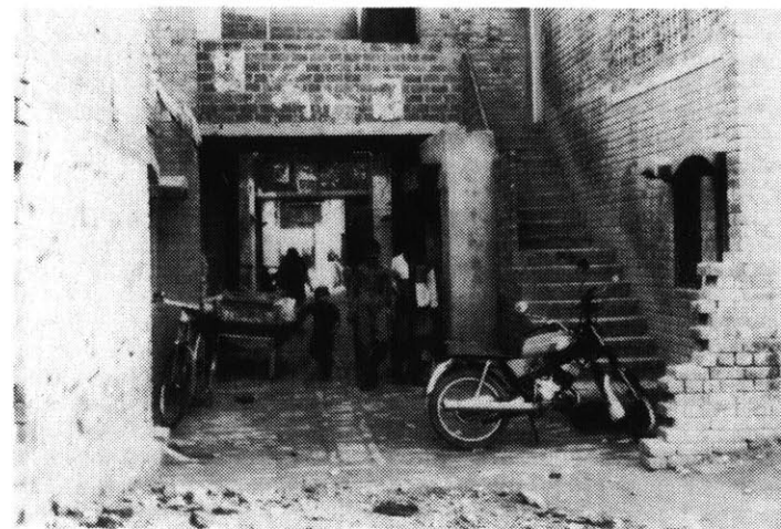
56. The streetscape, with interlocking and overlapping forms; and external vertical circulation.
