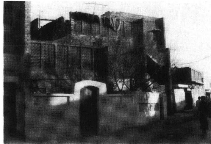
40. Angoori Bagh Scheme from the western encircling roads.
