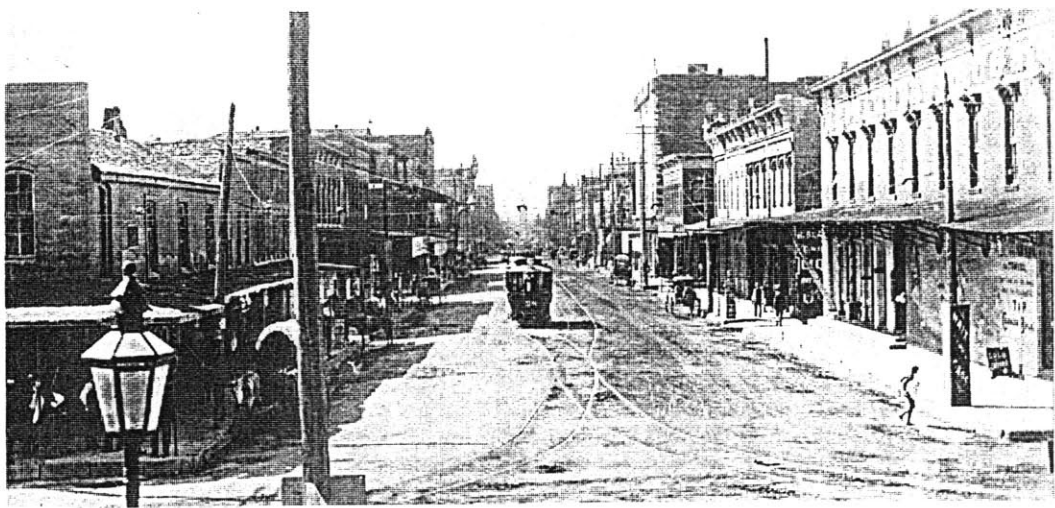
19. 1976 Street Car Service South View Down Main Street
