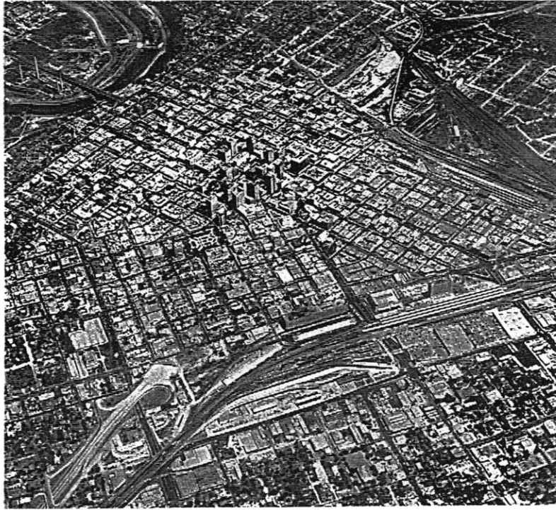
29. 1956 Existing View of CBD Traffic Before Gruen Plan
