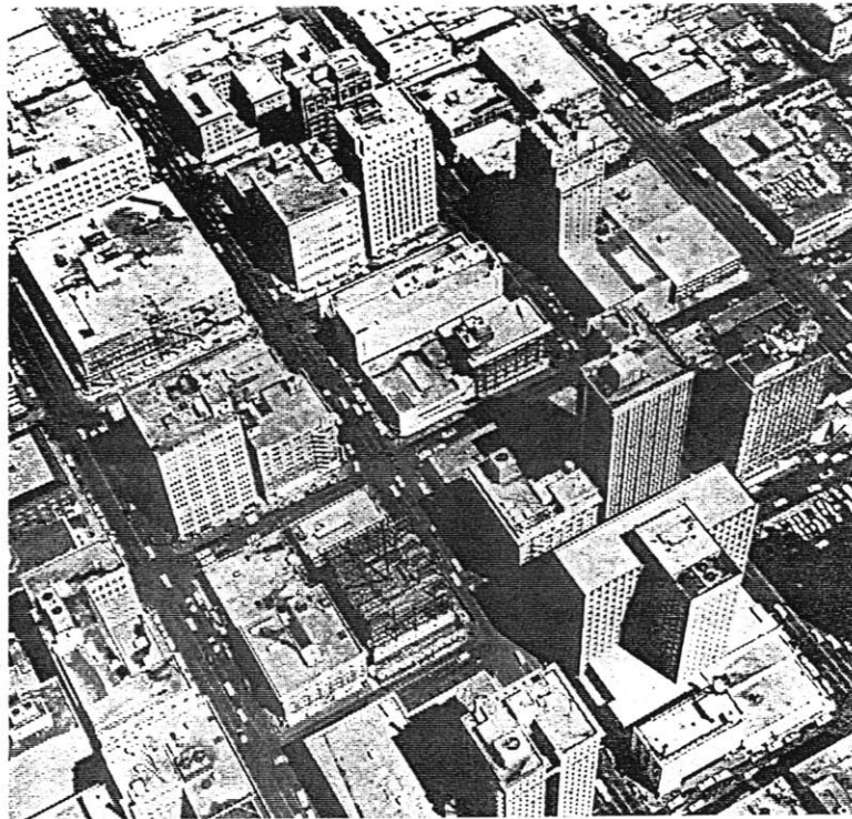
31. 1956 Existing Closer View of CBD Traffic Before Gruen Plan
