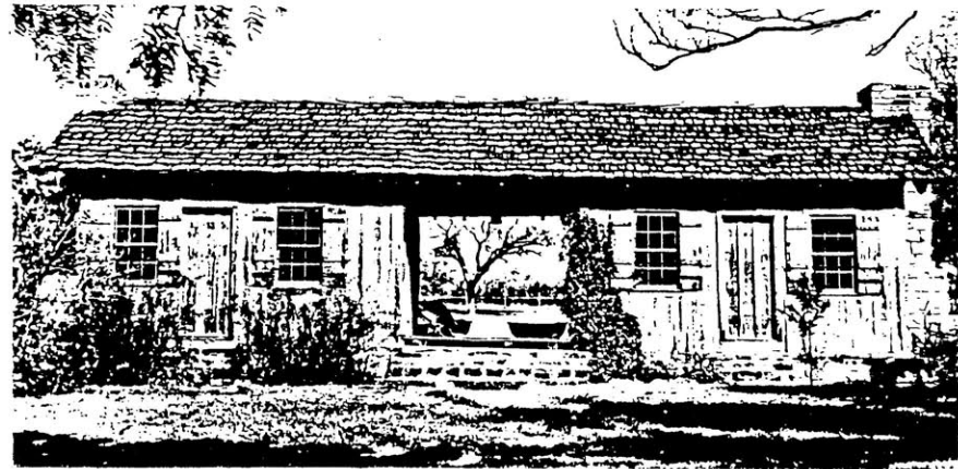
Dogtrot House. Source: Alexander,D.B. Photographs by Webb,T. . Texas Homes of the Nineteenth Century . Austin; University of Texas Press. NA7235.T4.A375 1966.
