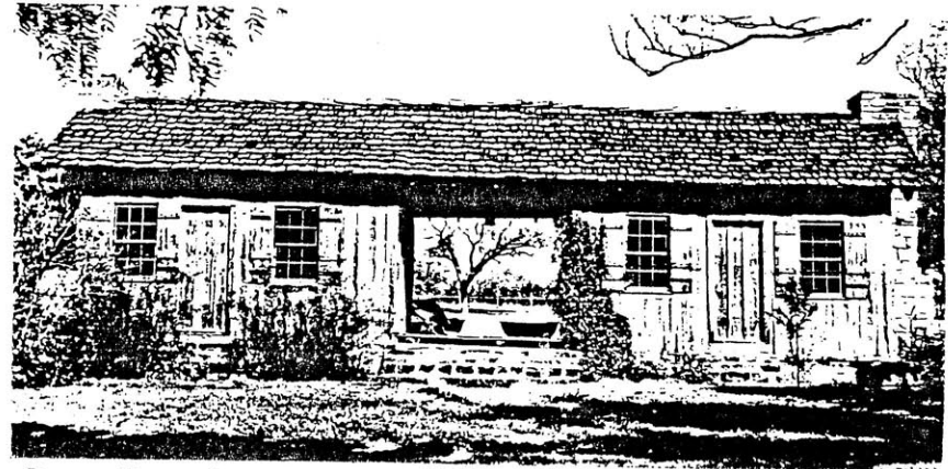
Dogtrot House. Source: Alexander,D.B. Photographs by Webb,T. . Texas Homes of the Nineteenth Century . Austin; University of Texas Press. NA7235.T4.A375 1966.
