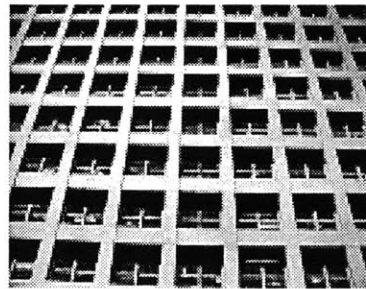
Figure 31: Typical Parking Garage in Downtown
