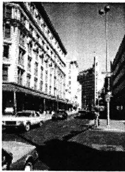
Figure 17: Street View of Urban Collector
