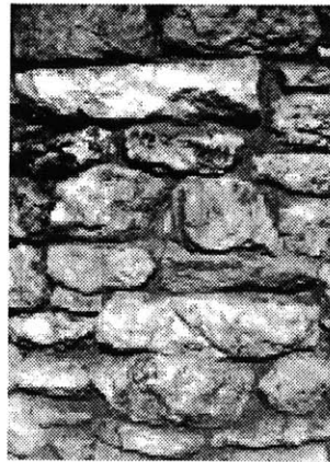
Figure 58: Texture of Local Walls
