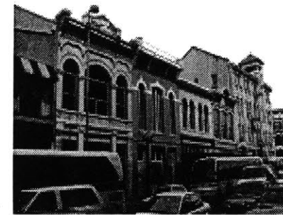
Figure 42: Typical Buildings along Commerce Street
