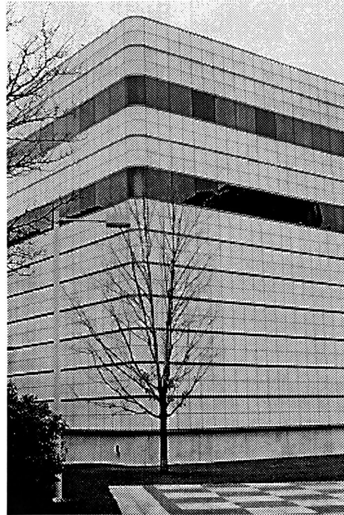
Figure # 11 Existing Wiesner Building, exterior curtain wall
