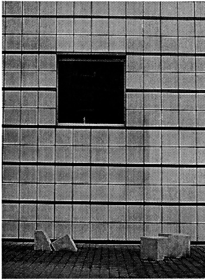
Figure #13 Existing Wiesner Building, curtain wall detail of single window
