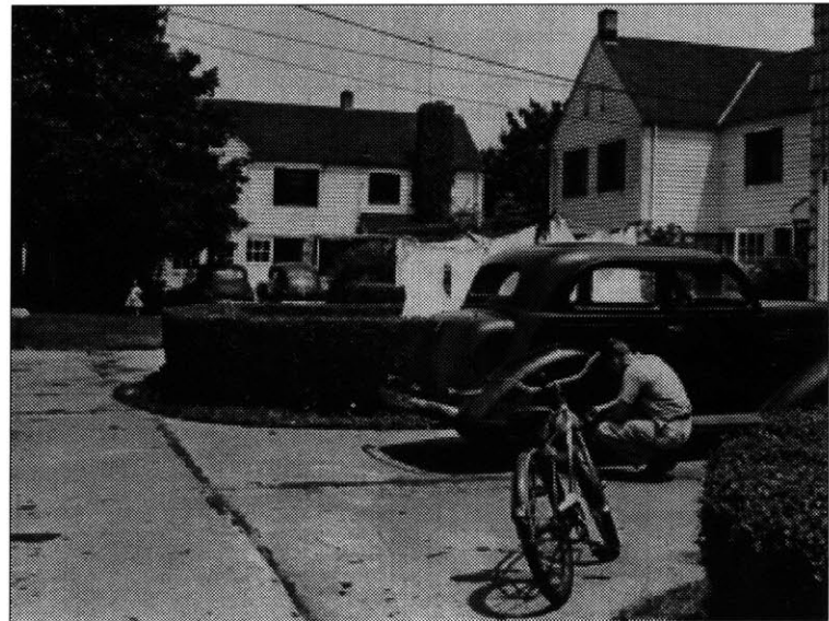
figure 47.2 Service road side of house cluster.
