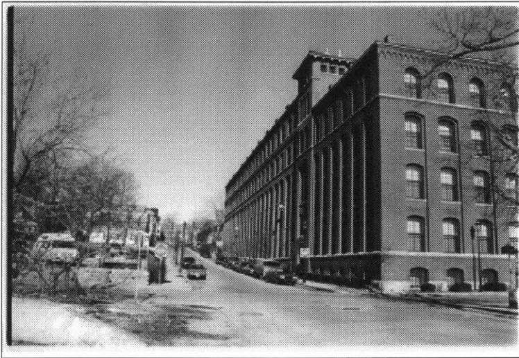
figure 24.1 Renovated Industrial Mill at Center of Site
