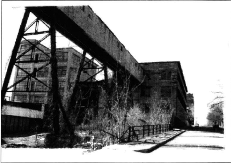
figure 9.1 Abandoned Industrial Buildings near Railroad Bed.
