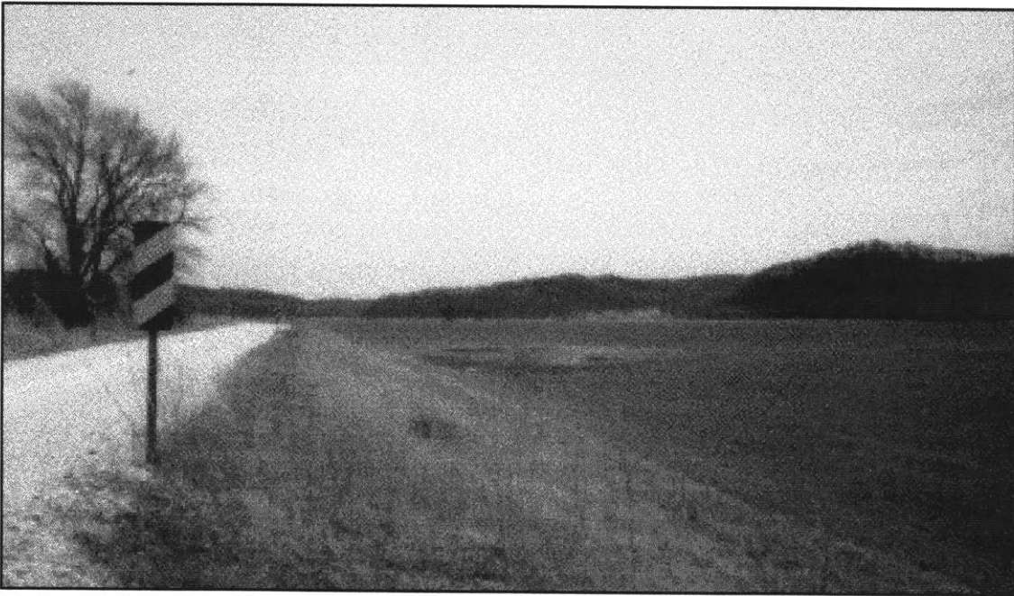
10 Small scour hole behind the new levee near Wilton, Missouri (Author, March 1996)
