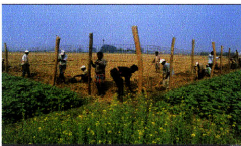
Fig. 22 Agricultural land being sealed off for land use conversion-setting it up for an SEZ
