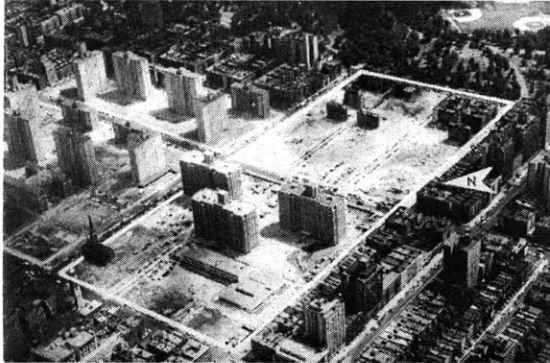
West Park housing estate under construction, New York City. 1958
