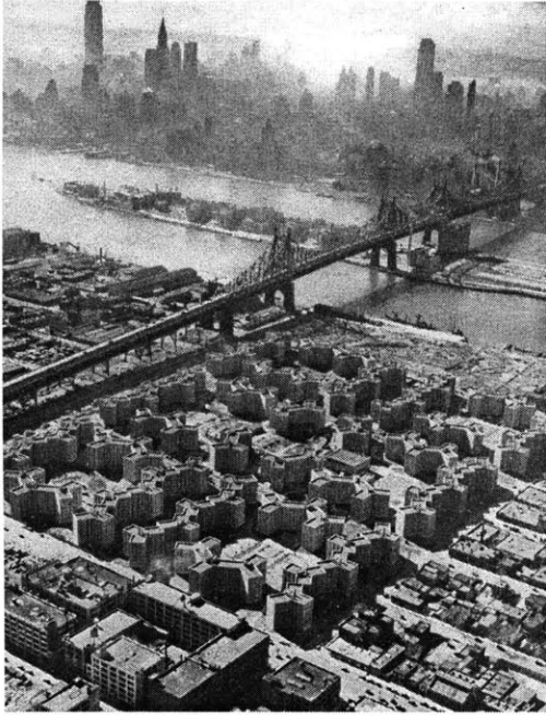
New York City public housing project, illustrated in Can Our Cities Survive? , Sert, 1942
