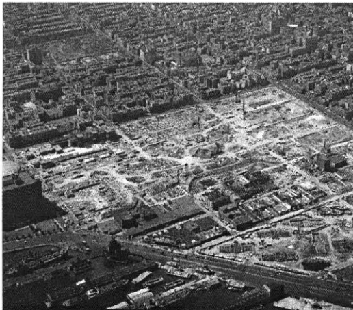
Stuyvesant Town under construction on slum clearance site, Manhattan, 1943
