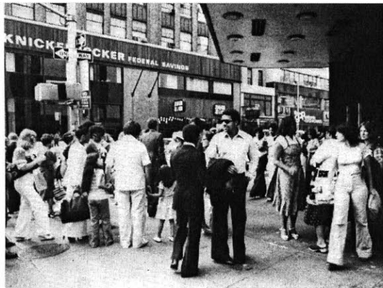
Midtown street corner, 1970's. from Whyte, Social Life of Small Urban Spaces
