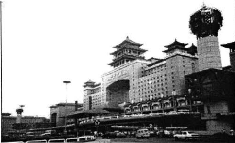
West Railway Station
