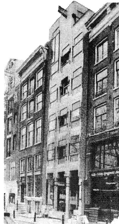
House and Offices, Amsterdam/Netherlands - Abel Cahen, 1971 Scale of the building is compatible with adjacent buildings. Certain dimensions are kept, the flatness of the façade plane is respected, the convention of using the ground level for public services is continued. Good points that the building introduces newly to the area are: façade material is consistent with the structural system used, structural system is exposed, balconies are inserted, there is another balcony on the top that makes use of the roof level.
