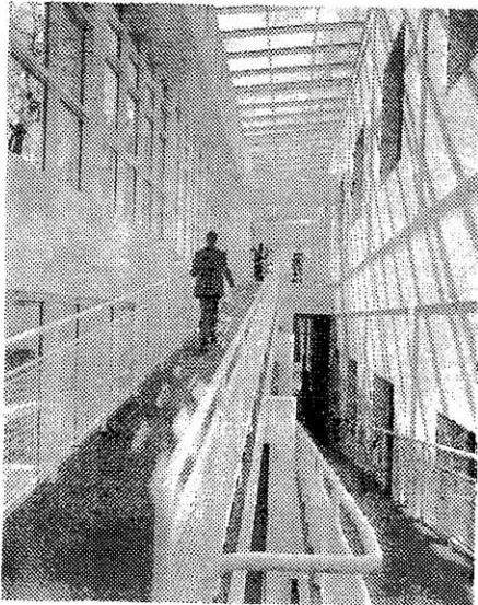
Museum for the Decorative Arts, Frankfurt/Germany - Richard Meier Frankfurt Museum is a good reference for ramps that are located parallel to skin of the building and that are used efficiently for any kind of access.
