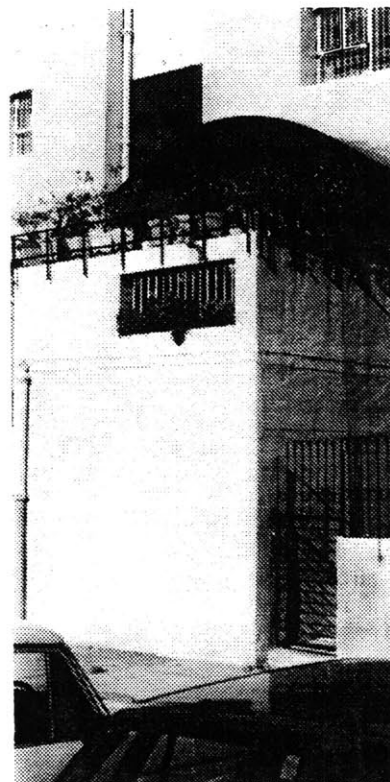
[43] Terrace with partial roof installed
