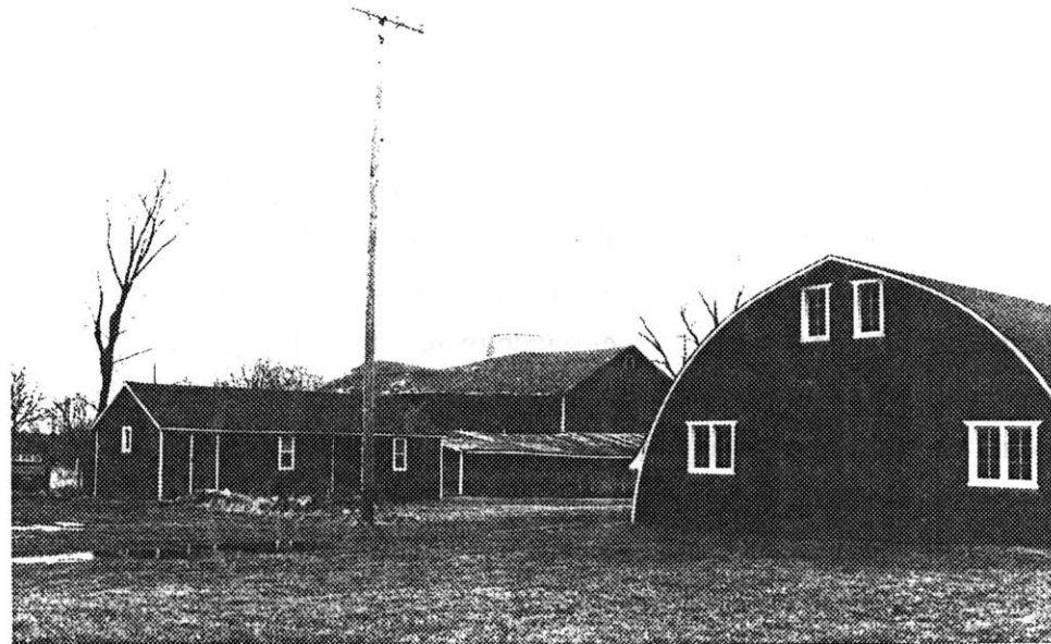
Figure 36: These are barns located on the Plymouth site. They are owned by the Islamic Center of America. The one on the left is being renovated and will be used for congregation social functions. By doing this, the planning committee wants to get members of the congregation motivated and used to traveling the distance to reach the site. The planning committee hopes to lessen the resistance to the site based on its distance from Dearborn.
