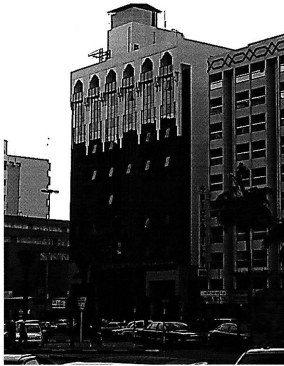
Fig. 19D Habib Bank Building- Baniyas Square
