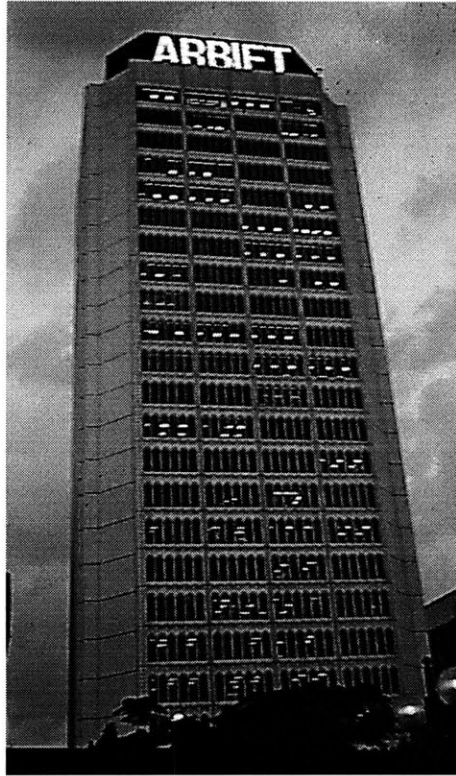
Fig. 15D ARRIFT building
